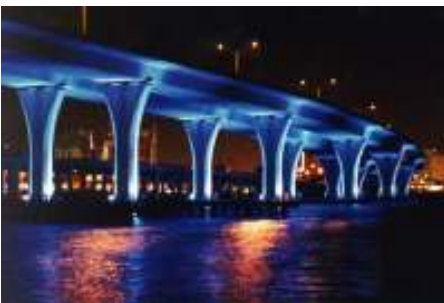
Merrill Barber Bridge, Vero Beach, Florida
