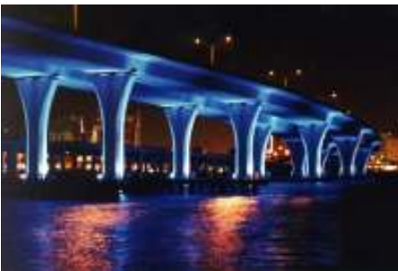
Merrill Barber Bridge, Vero Beach, Florida
